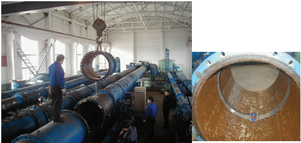
Figure 2. Test pipe line and installation of the V-ADCP transducer
