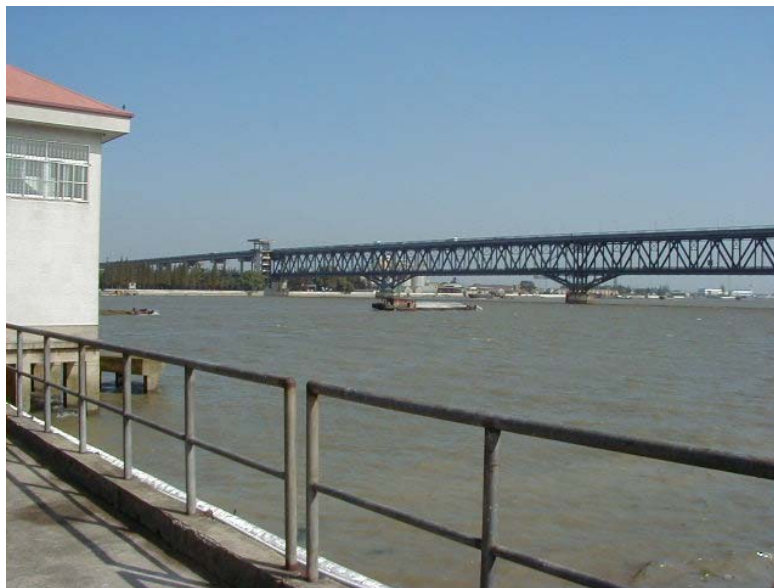
Figure 12 Huangpu River at Songpu Bridge Site, Shanghai, China
